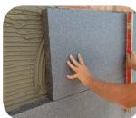
Once the plates have been placed with the joints intercalated and with the dry mortar (24 hours), they will be drilled for the placement of the fixing plug.
