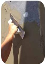
After 24 hours approx. the surface will be regulated and then with the fresh paste the mesh will be spread across the entire surface.
