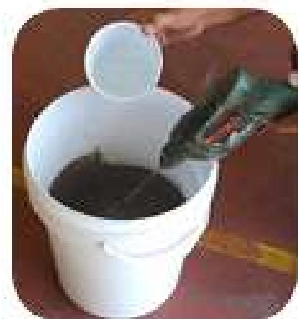
Mix the components **A + B** with a low revolution whisk until obtaining a perfect homogenizing.
