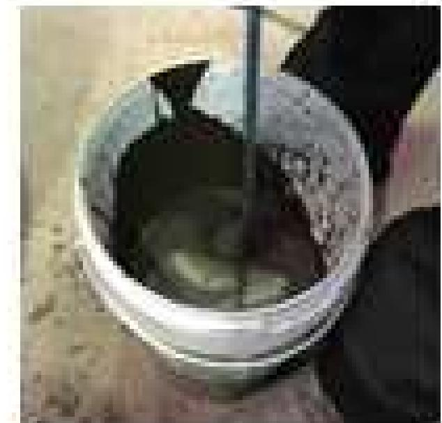
Mix components **A+B** with a whisk at low speed for at least 2 minutes, add component **C** (powder) and mix for approx. 1 minute, until perfectly homogenised.
