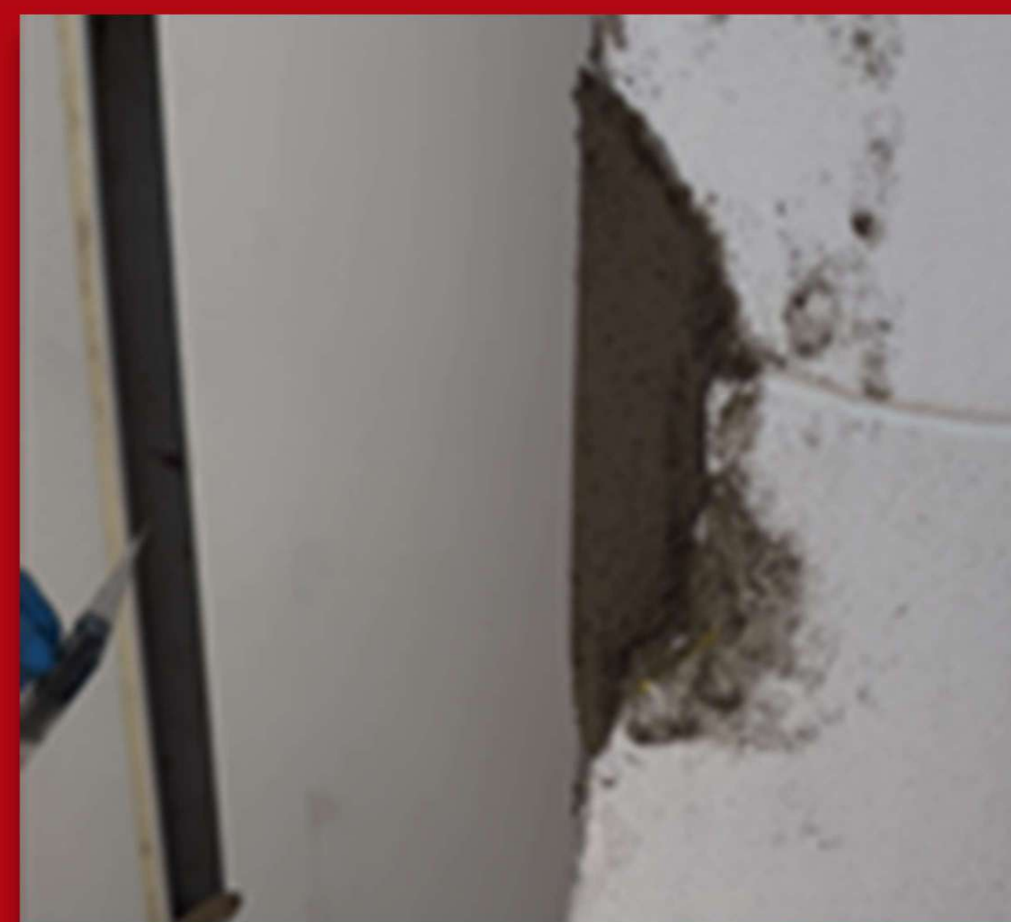
8. Finished to be coated.
