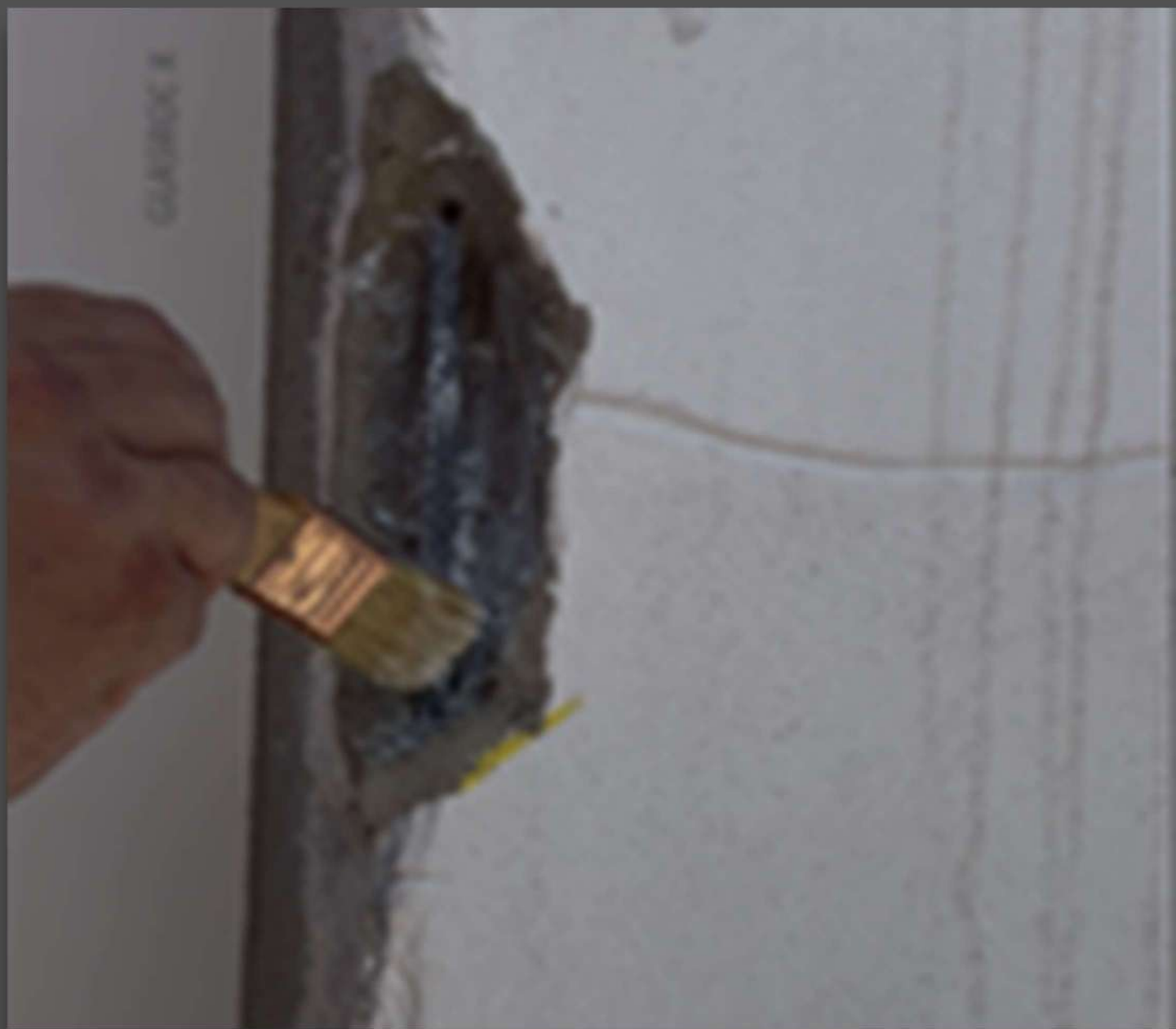
4. Can be applied over concrete as a bonding bridge.
