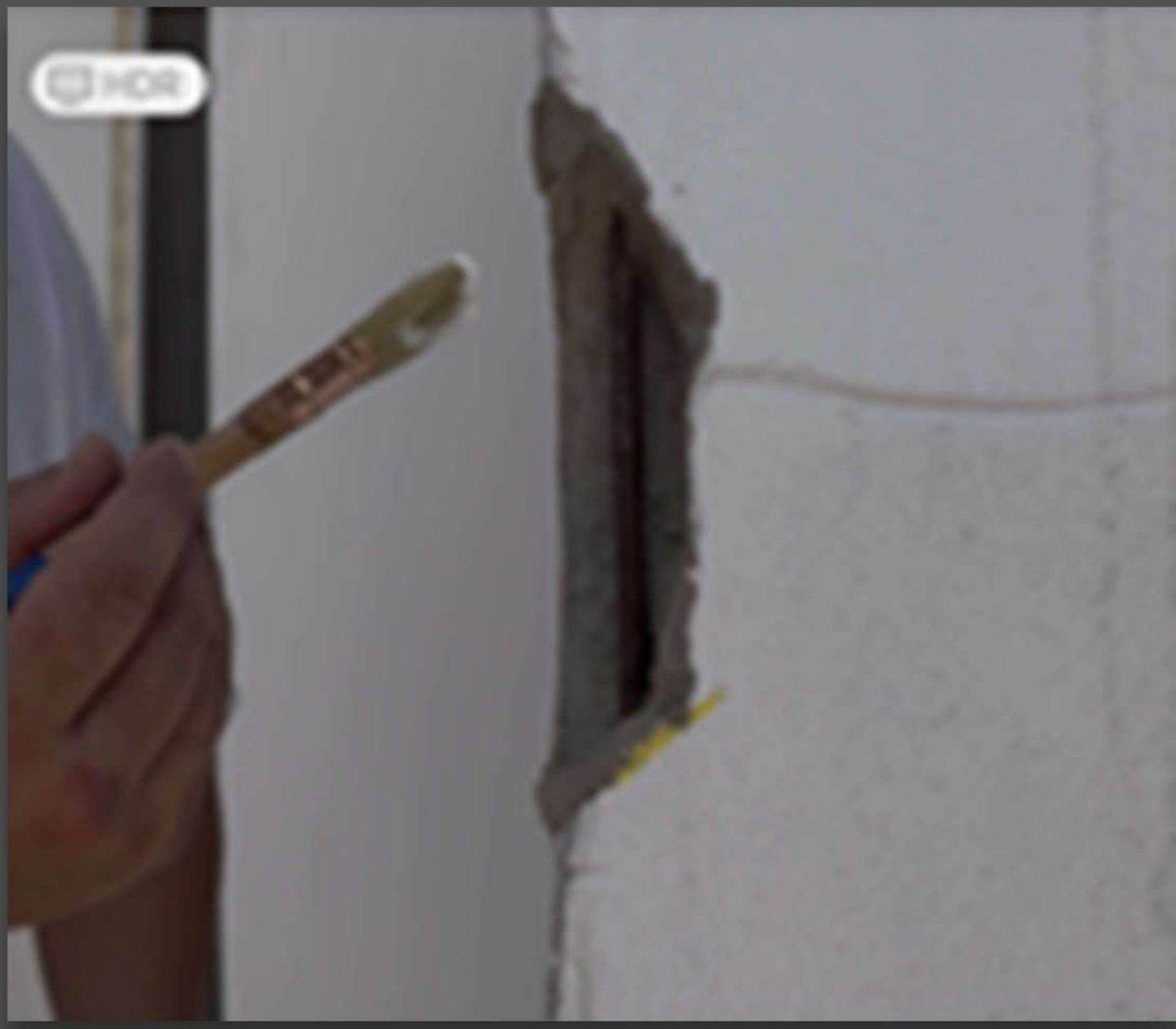
2. Clean support, no rust or chips.
