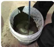
Mix components **A + B** with a mixer at low revolutions for at least 1 minute, until a perfect homogenization is obtained.
