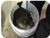
Mix components **A + B** with a whisk at low speed for at least 2 minutes, add component **C** and mix for a further 2 minutes, until a perfect homogenization is achieved.
