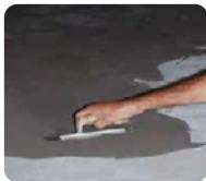
The application can be made with a steel or rubber trowel.
