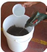
Mix the components **A + B** with a low revolution whisk until obtaining a perfect homogenizing.
